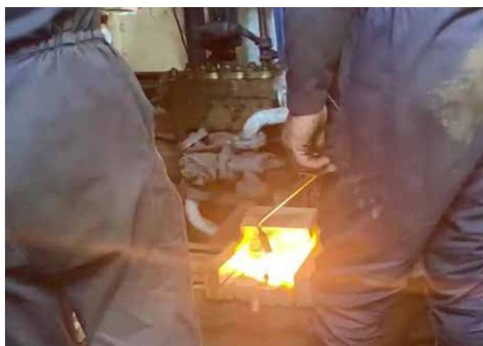
to remove the old rivet, prepare the hole and trial fit the new one, heat it up, insert it in the hole and round both ends off using pneumatic hammers. You'll have seen the process in old documentaries about building liners, I expect.
