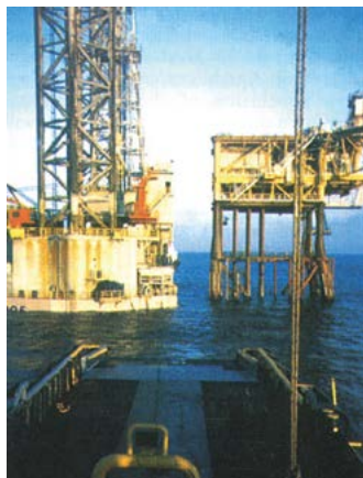
Towing the rig away from the platform
